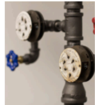
Bottom right Floor Lamp details Pipes and industrial objects salvaged from BFGoodrich steam plant Whiskertin Lighting
